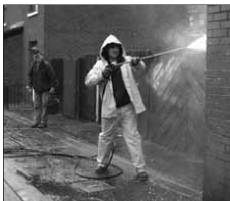
Housing Executive power wash graffiti
